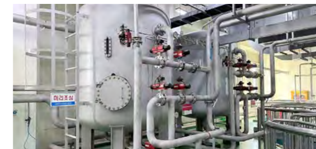
Celltrion Pharm Wastewater Treatment Plant
